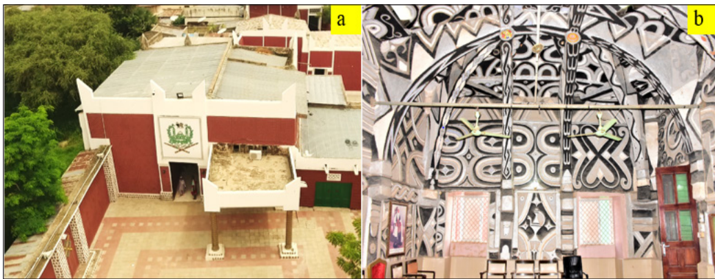
Figure 7. (a) Aerial view of the monumental guest-chamber Soron Giwa , showing the zinc roof sealing the mud roof and then cladded with the masonry wall; (b) The preserved interior of soron Giwa in its earthen form
